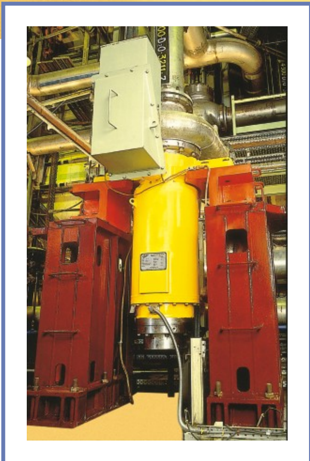
Kirloskar Canned Motor Pump (CAN 220) at Nuclear Power Corporation of India Ltd., Tarapore
