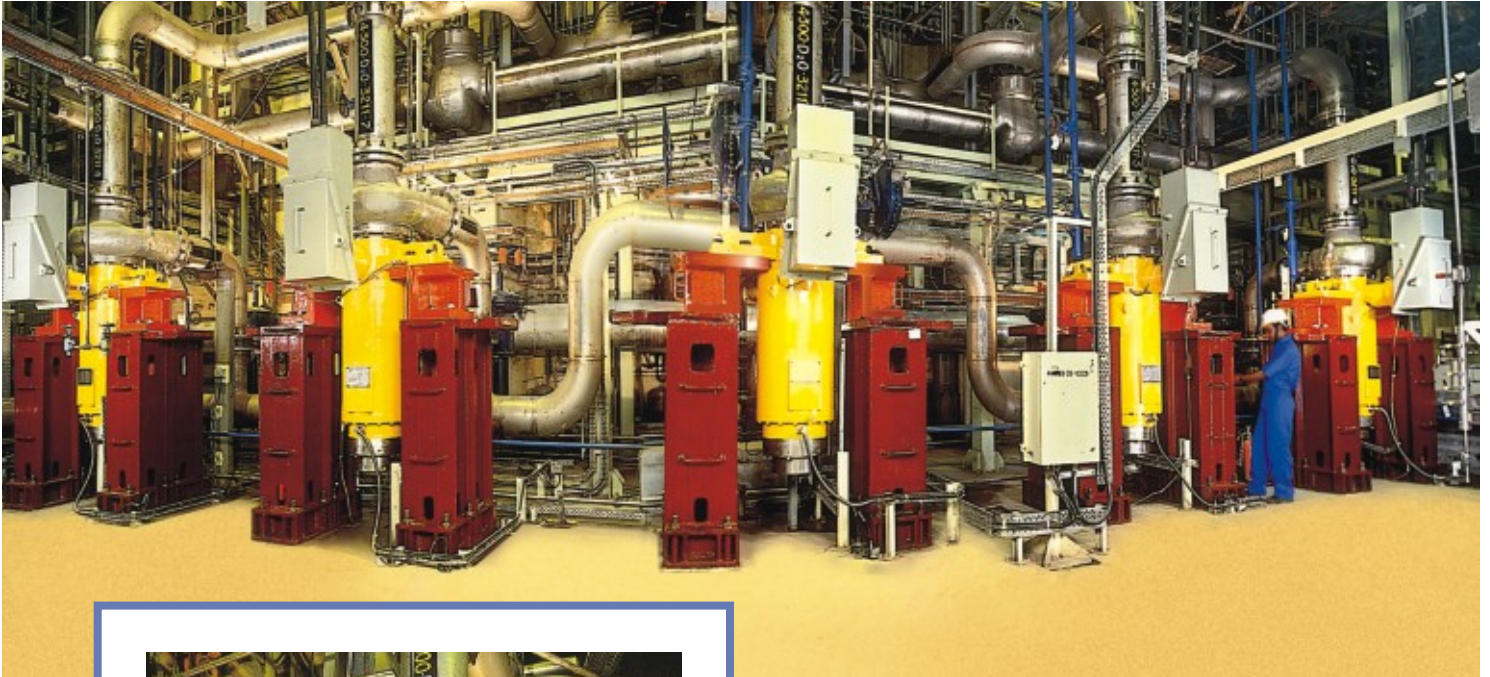
Kirloskar Canned Motor Pump (CAN 220) at Nuclear Power Corporation of India Ltd., Tarapore
